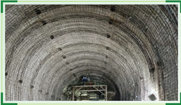
T11P1-Overt reinforcement binding work is in progress
