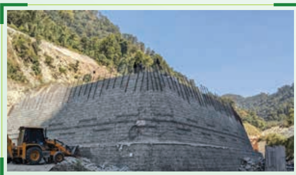
Construction of RE Wall at Rangpo Yard
