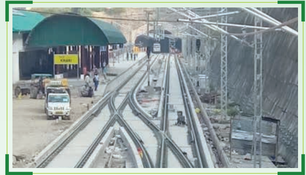
Thick web canted turnouts with weldable crossings on ballast less track
