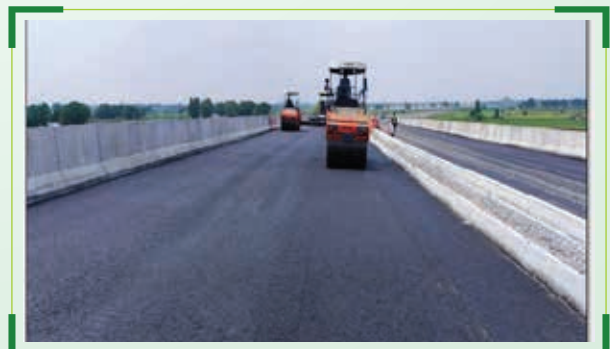
DBM laying , Gurgaon Rewari Highway Project
