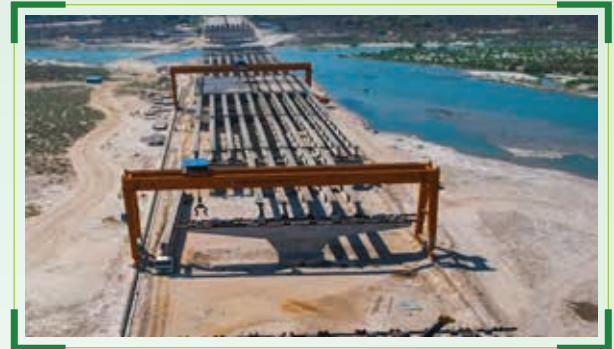
Girder Launching & Sub Structure WIP at Major Bridge, Haridwar Bypass Project
