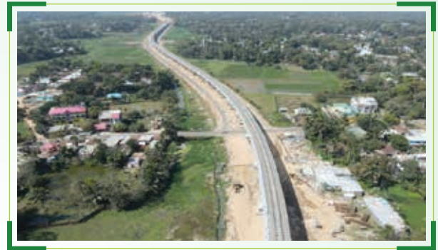
Viaduct, Agartala Akhaura Rail Link Project
