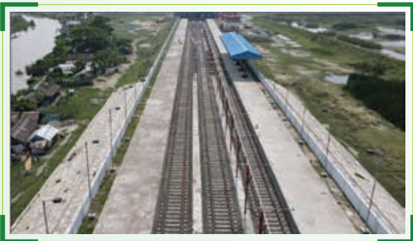
Mongla Station Yard
