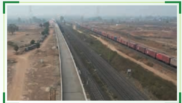
Katni Grade Separator Project
