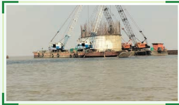
Well Foundation in Progress
