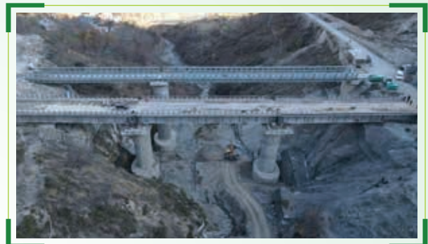
Bridge no. 138, USBRL Project
