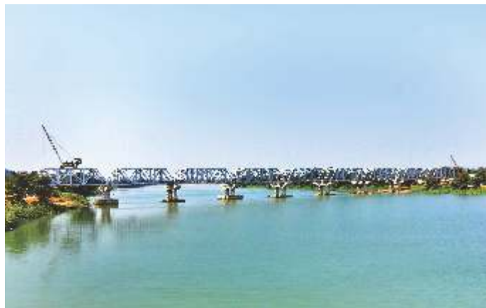
Railway bridge No. 17, Chhattisgarh
