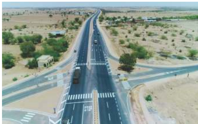
Bikaner-Phaludi Highway Project
