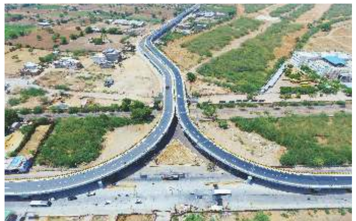
ROB at Jodhpur, Rajasthan
