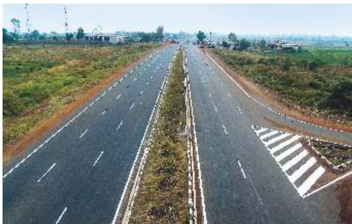
Shivpuri - Guna 4 Lane Highway Project
