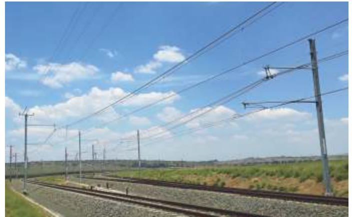
Railway Electrification work, Majuba, South Africa
