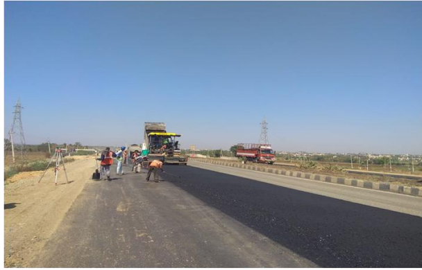
DBM Laying (Lane-2) at 329+500 LHS
