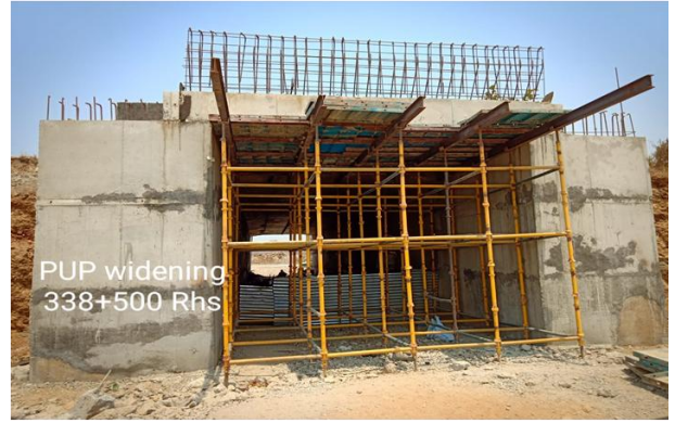
338+500Rhs PUP widening
