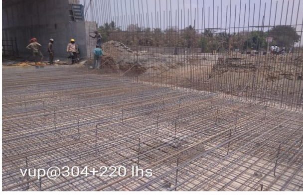
304+220 VUP Reinforcement in Progress
