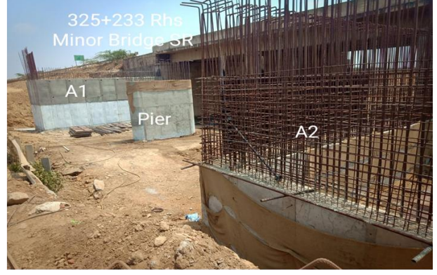
325+233 RHS Minor Bridge
