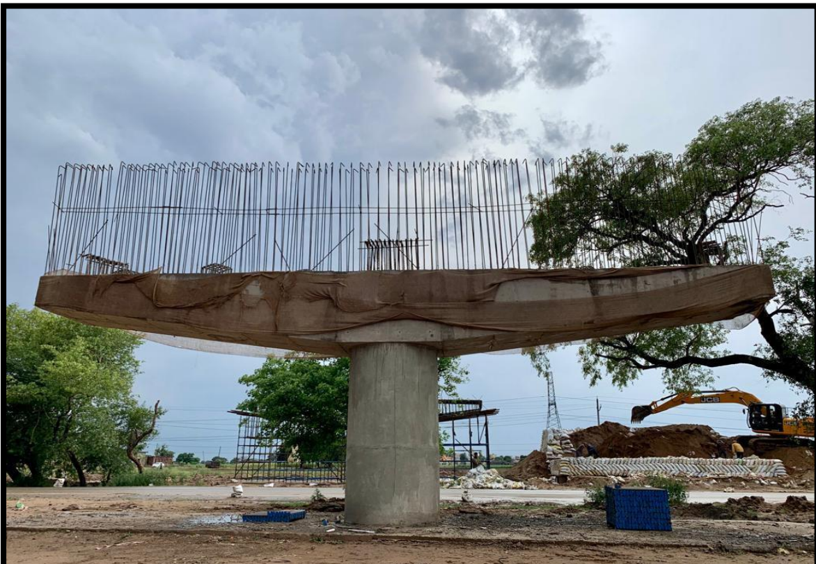
Abutment (A2) of Flyover @ Ch:9+270
