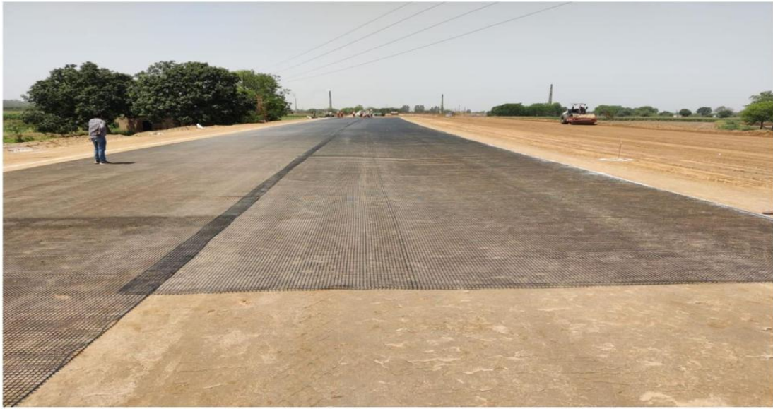
GEO-GRID LAYING @ Chainage 81+850 to 82+100
