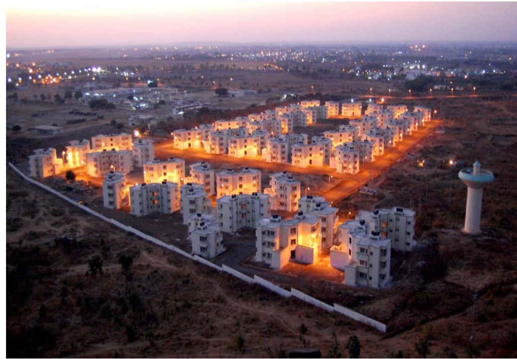
Married Accommodation Project
