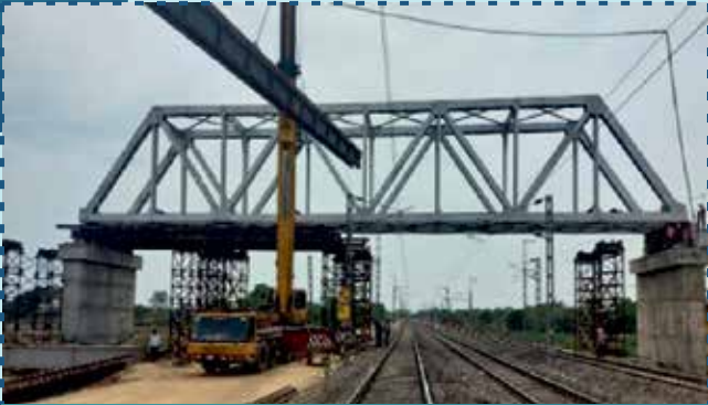
RoR Launching Bridge 5A near Kharsia, Chhattisgarh East Rail Corridor
