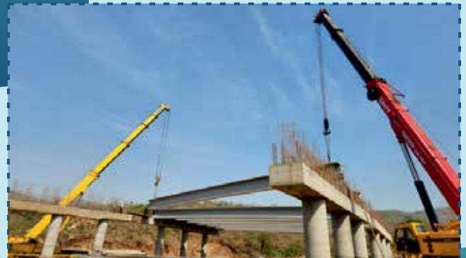
UHPFRC Girder Erection, Bhoj Morbe Expressway Project
