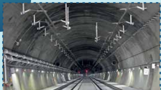
ROCS Erection in Tunnel T-50, USBRL Project
