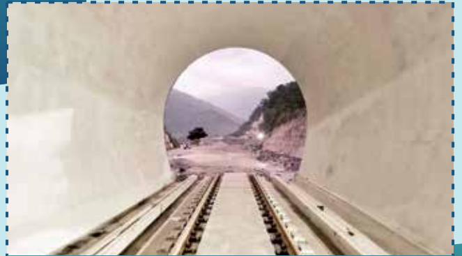
T14 BLT Work, Sivok Rangpo New Rail Line Project
