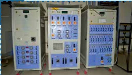
Integrated Power Supply, Moradabad S&T Project
