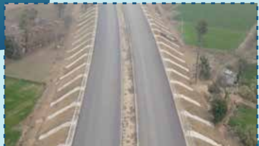
DBM Work with Side Slope Protection @ Ch 68+100, Ludhiana Rupnagar Highway Project
