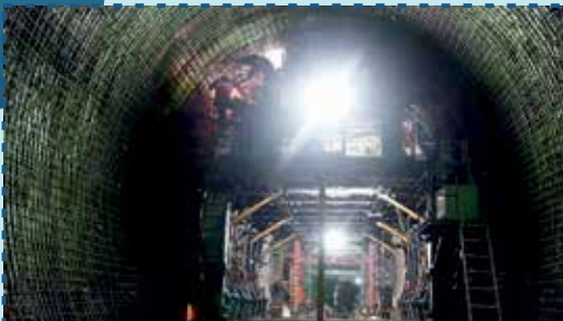
Lining is in progress, Sivok Rangpo New Rail Line Project
