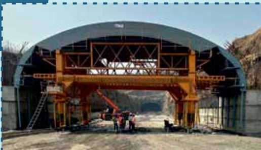
Cut & Cover Gantry Erection, Bhoj Morbe Expressway Project
