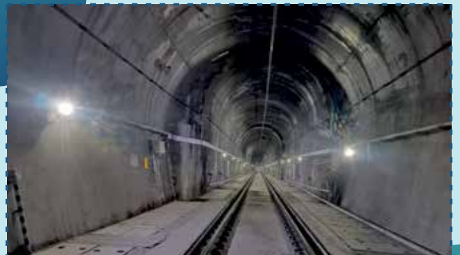
T-52 D-SHAPE & H. SHOE, USBRL Project
