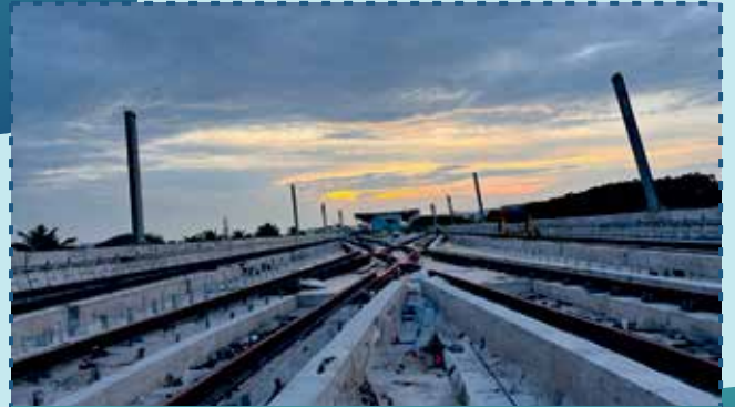
Scissor Cross Over with Track centre 12 M, Chennai Metro Rail Project
