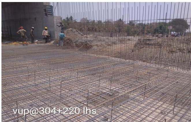
304+220 VUP Reinforcement in Progress
