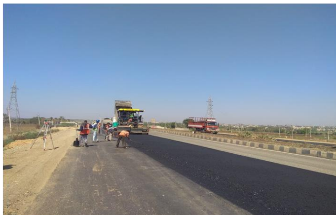
DBM Laying (Lane-2) at 329+500 LHS
