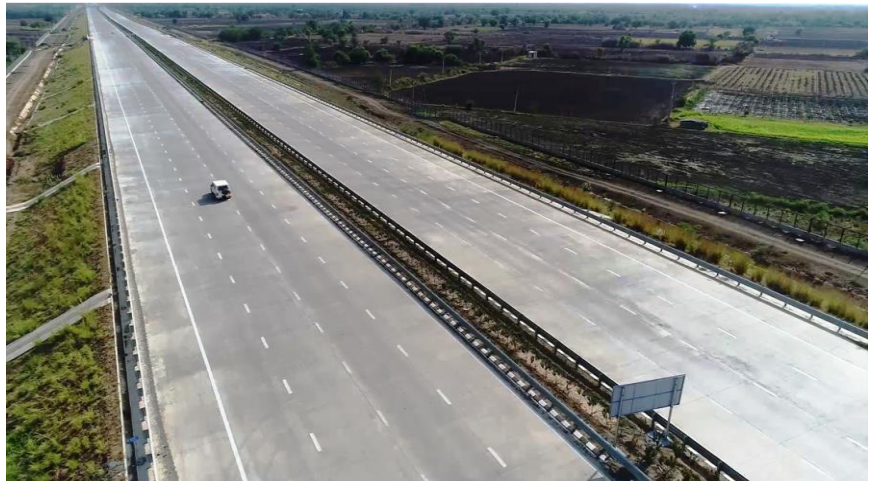
Vadodara Kim Expressway Project
