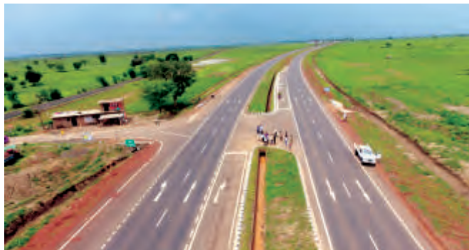
Shivpuri-Guna Four Lane Highway project
