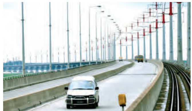
Dual gauge Railway line Bangladesh
