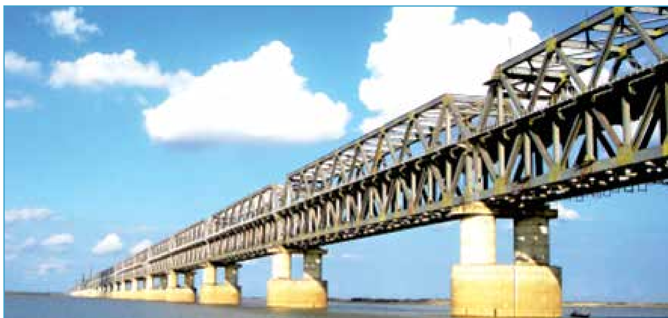
Rail- cum-Road Bridge at Patna, Bihar
