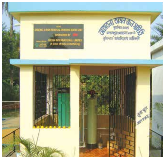
Water Treatment Plant at North 24 Parganas (WB)
