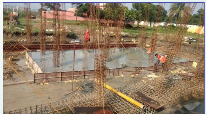
CONSTRUCTION SITE, LPAI Project- Jogbani, Bihar
