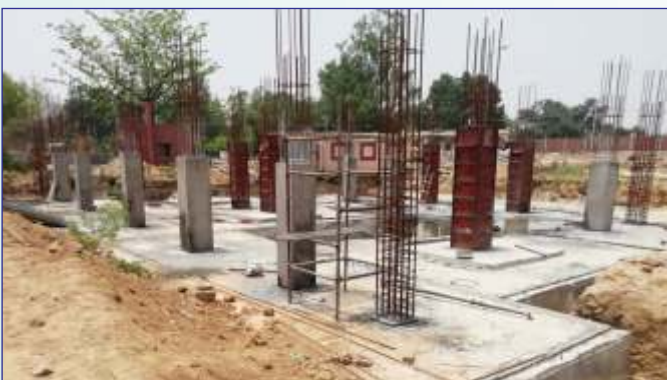
CONSTRUCTION SITE, LPAI Project- Attari, Punjab
