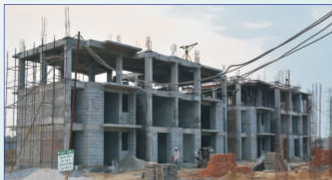
SHRI VISHWAKARMA SKILL UNIVERSITY - CONSTRUCTION SITE
