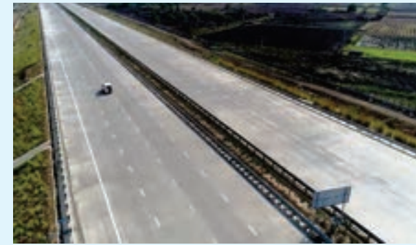
Vadodara Kim Expressway Project
