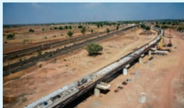
Katni Grade Separator Project
