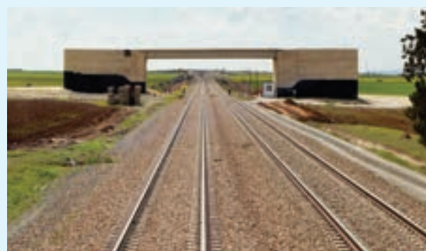
ROB under construction above the completed double track, Algeria
