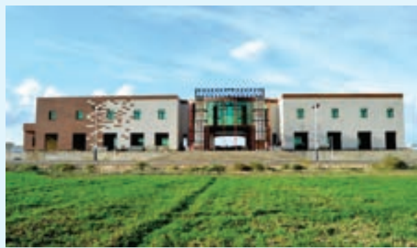
Relizane Station Building at Algeria
