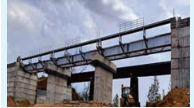
Composite Girder - Katni Singrauli Rail Doubling Project
