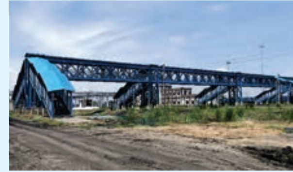
Nabinagar Super Thermal Power Project
