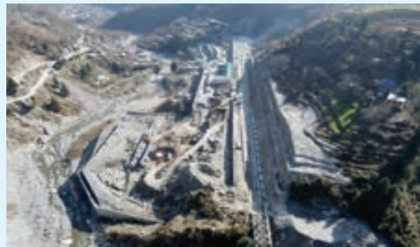
Aprinchala Yard in Udampur Srinagar Baramulla Rail Link Project
