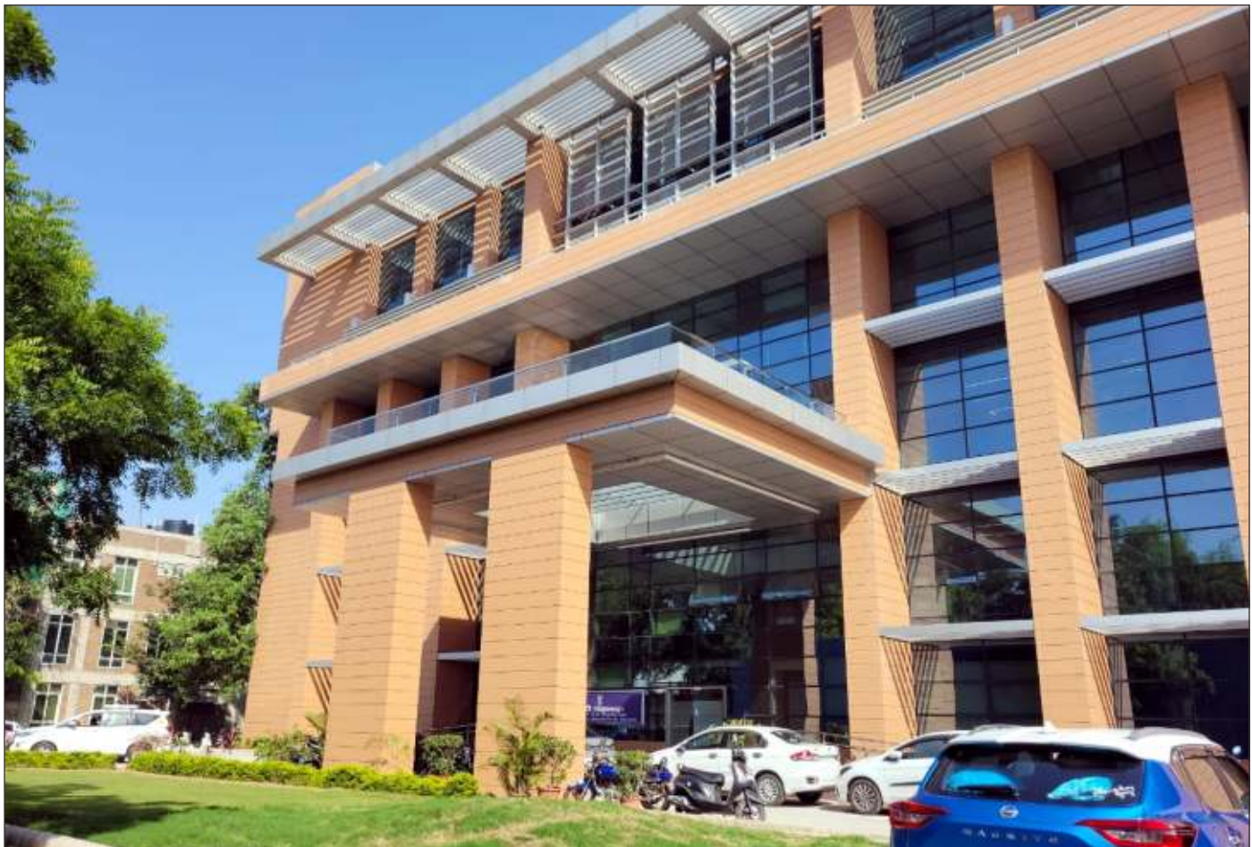
Construction of new State of Art Building of Development of Science & Technology at Technology Bhawan, New Mehrauli Road, New Delhi
