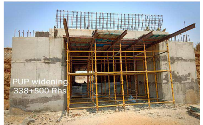
338+500Rhs PUP widening
