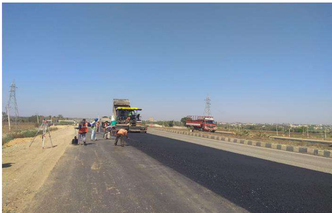
DBM Laying (Lane-2) at 329+500 LHS
