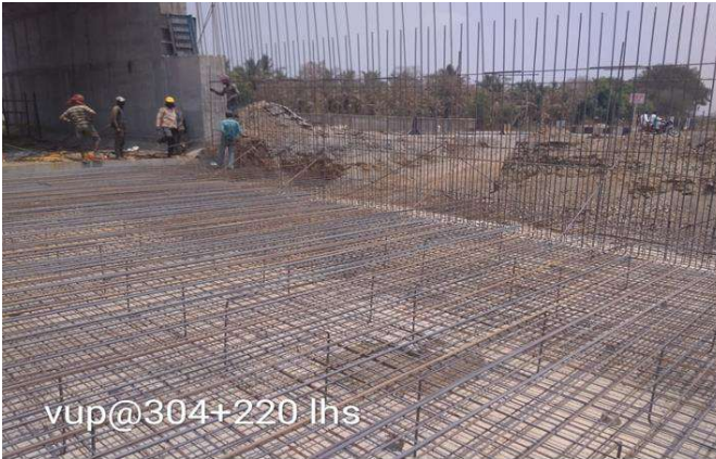
304+220 VUP Reinforcement in Progress
