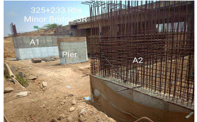
325+233 RHS Minor Bridge
