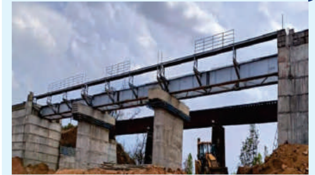
Composite Girder - Katni Singrauli Rail Doubling Project
