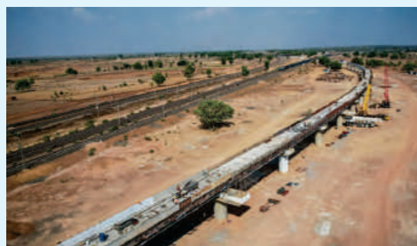
Katni Grade Separator Project
