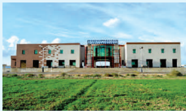
Relizane Station Building at Algeria
