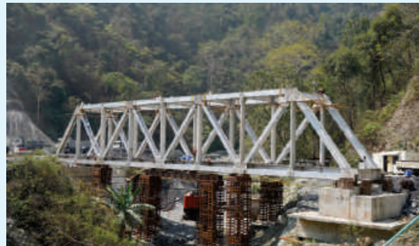
Erection of OWG at Bridge No 04 - Sivok Rangpo Railway Line Project
