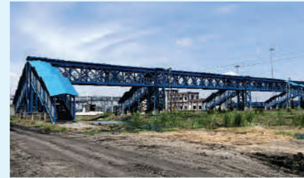
Nabinagar Super Thermal Power Project
