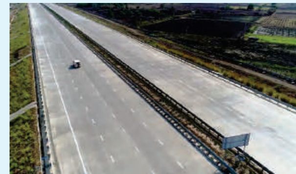
Vadodara Kim Expressway Project
