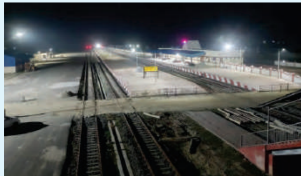
Nepal Custom Yard - Jogbani Biratnagar Project
