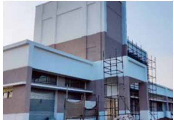
DFC Station Building at Ancheli (Gujarat).
