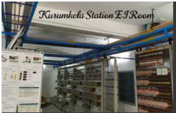
CERL – I Electrification Work
