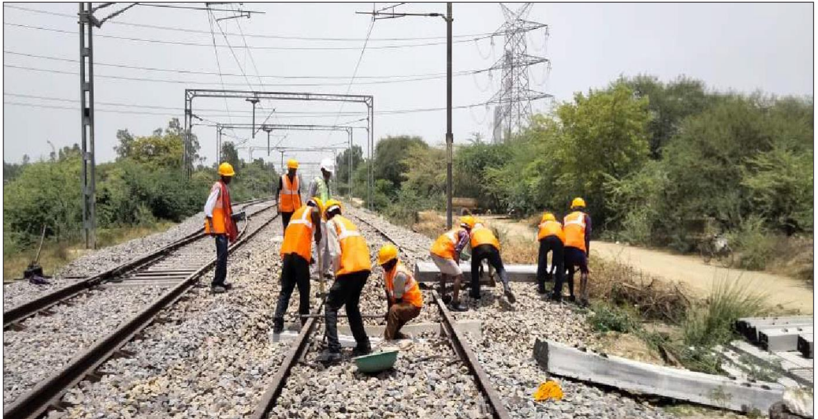
Progress for Replacement of CST-9 Sleepers with PRC Sleepers at NTPC,
